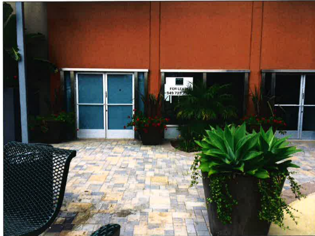
FRONT ENTRANCE TO UNIT F
