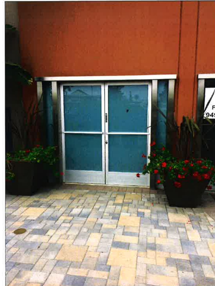
FRONT ENTRANCE TO UNIT F
