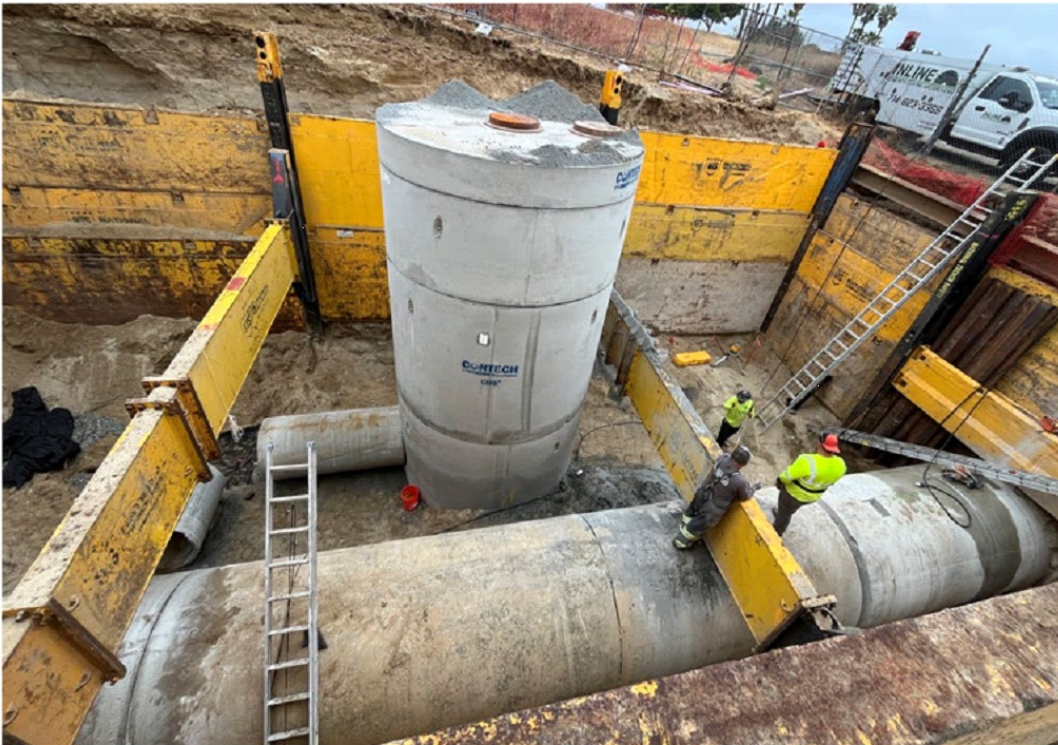
Newly installed Hydrodynamic Separator Unit
