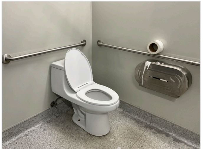
TOILET STALL OVERVIEW
