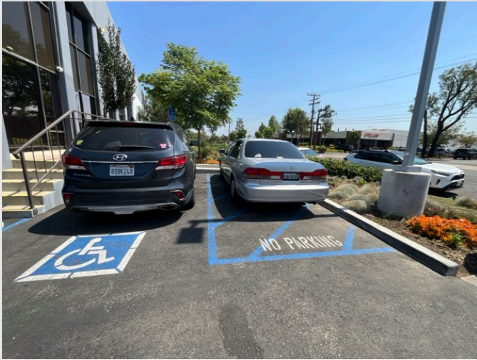
OVERVIEW OF ACCESSIBLE PARKING AREA
