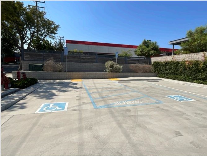
OVERVIEW OF ACCESSIBLE PARKING AREA
