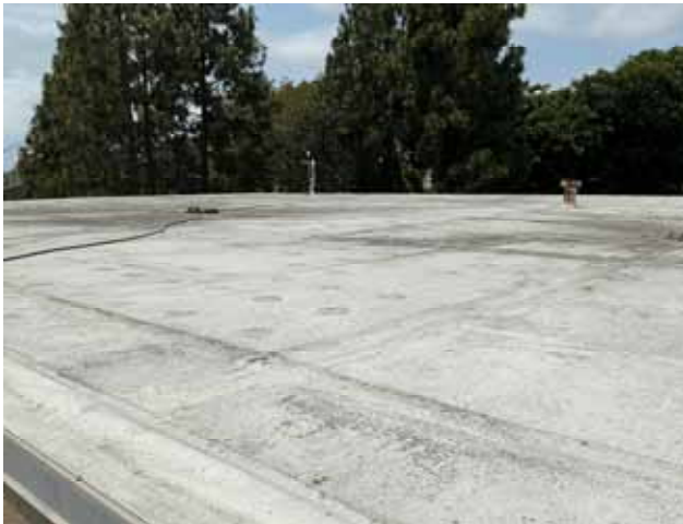
9 - PRIMARY ROOF OVERVIEW
