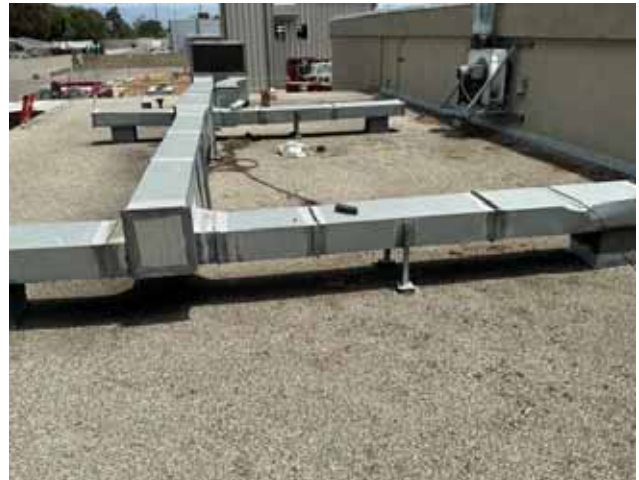
10 - SECONDARY ROOF OVERVIEW
