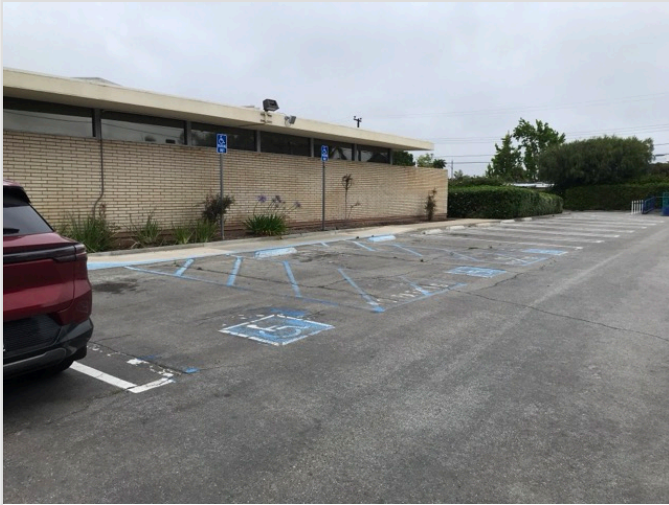
OVERVIEW OF ACCESSIBLE PARKING AREA
