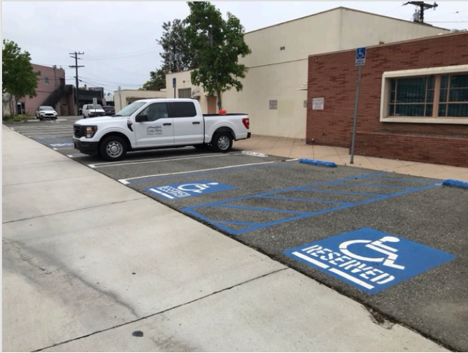
OVERVIEW OF ACCESSIBLE PARKING AREA
