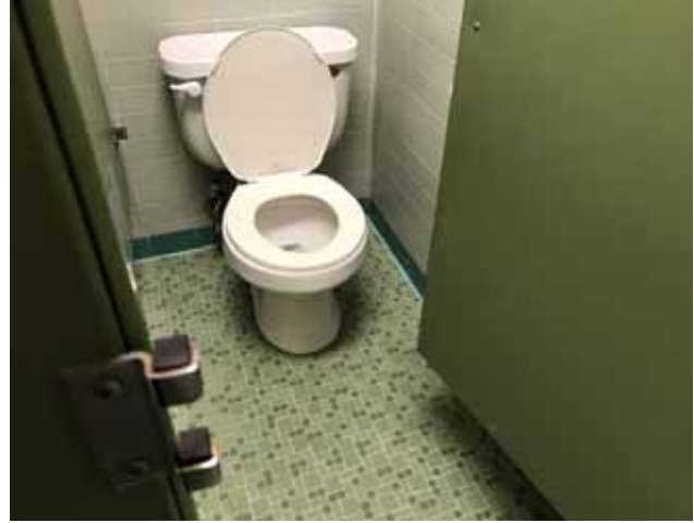
14 - TOILET STALL OVERVIEW
