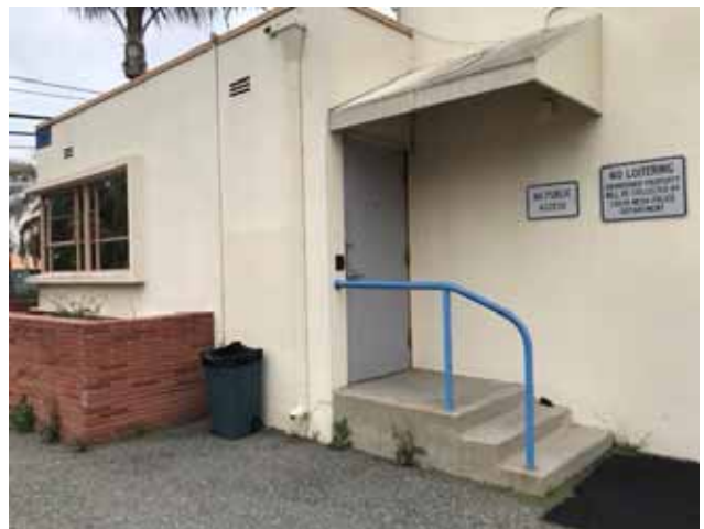
6 - EXTERIOR DOOR AND WINDOW
